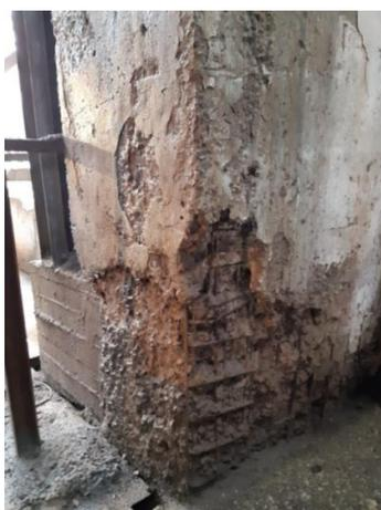
Fig. 7. The results of long-term destruction of concrete structures in the storage room for finished products under the influence of the environment
