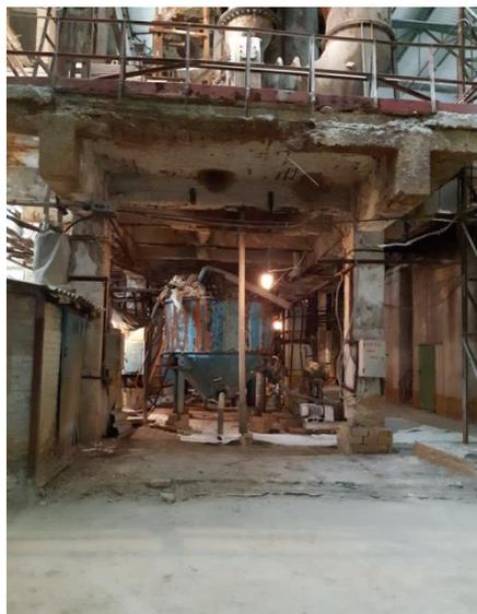
**Fig. 1.** Consequences of corrosion processes in the workshop for the production of titanium dioxide ( $\text{TiO}_2$ ) by the sulphate method
